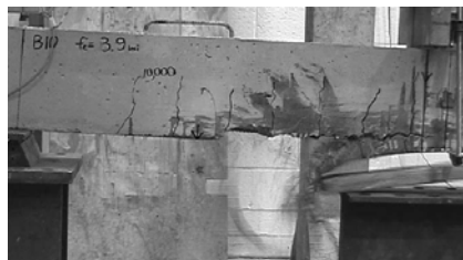
(b) Cover Delamination
