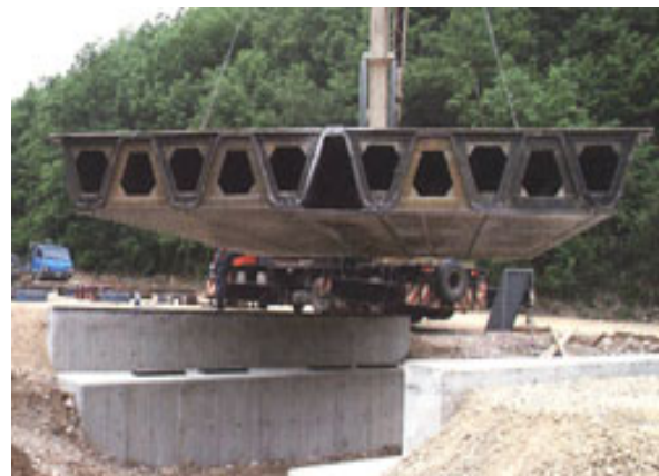
Fig. 18 Provincial road of Yeongweol - Gyunbuk (Composite material bridge)
