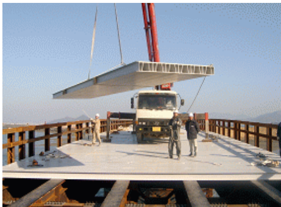
Fig. 17 Gwanhyang Harbor Bridge
