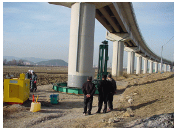
Fig. 10 Field test of FRP wrapping automation device
